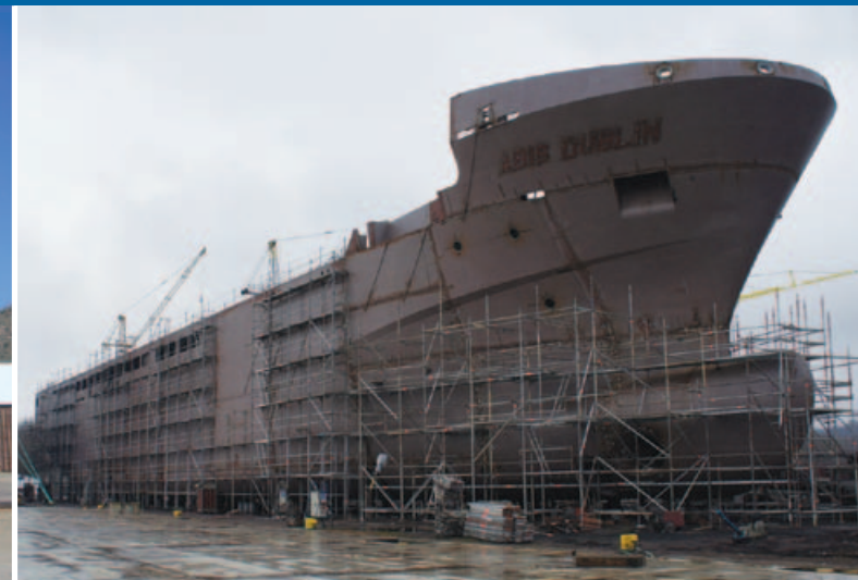
Left: Sunborn Hotelship under construction in Malaysia at Boustead Naval Shipyard.
