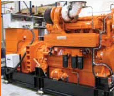
▲ DT709 with Mitsubishi S6R2 & Stamford HCM634
